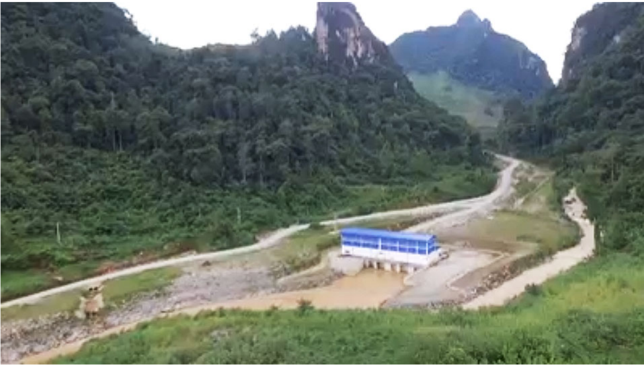
Nam Sana surge tank image below:
