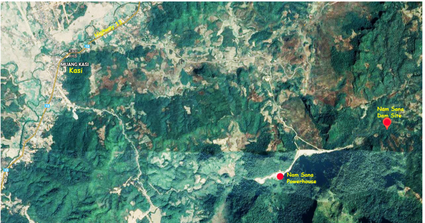
Nam Sana Powerhouse site image below:
