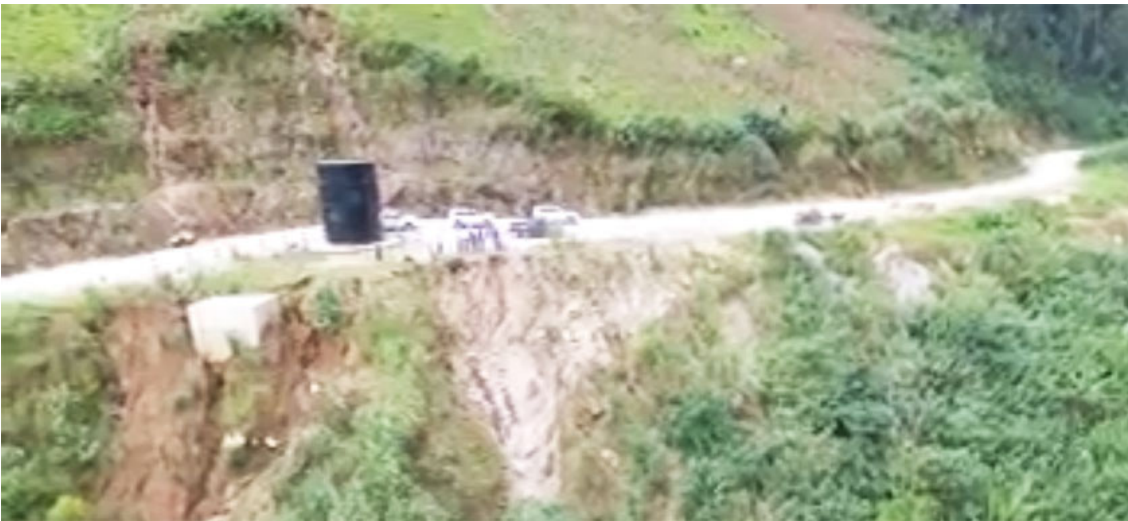
Nam Sana weir image below:
