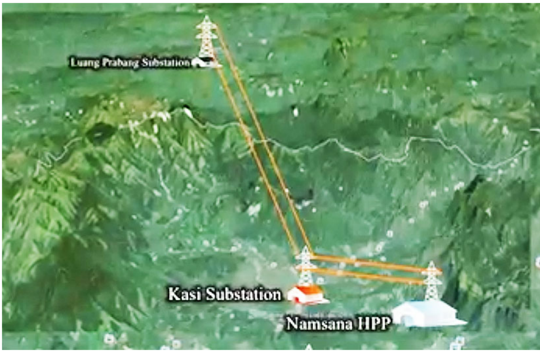
Nam Sana Powerhouse image below from Nam sana Facebook page - https://www.facebook.com/search/top?q=namsana%20hydro%20power%20plant :
